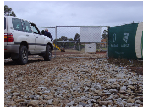
Figure 2.7.1 - Example of a stabilised, all weather access point.
