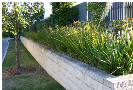
Figure 2.12.1 - Example of a retaining wall.
