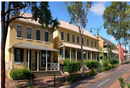
Figure 2.11.3 - Careful consideration shall be given to any development that has the potential to impact on items of heritage and their setting.
