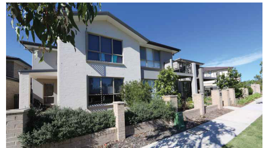
Figure 3.7.2.4 - An example of multi dwelling housing, with separate dwellings on each floor. (Source Dwelling Density Guide, NSW Planning & Environment, 2014)
