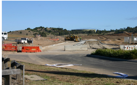
Figure 3.8.2 - Example of residential subdivision under construction.
