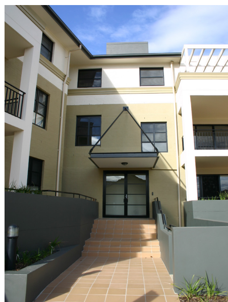
Figure 5.5.1 - Entry to residential flat building.
