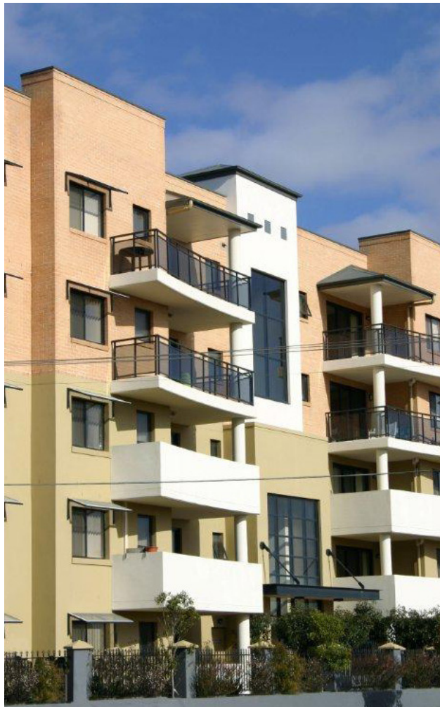
Figure 5.2.1 - An example of high density residential development.
