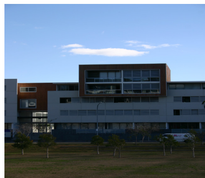
Figure 5.4.1 Example of contemporary residential flat building.
